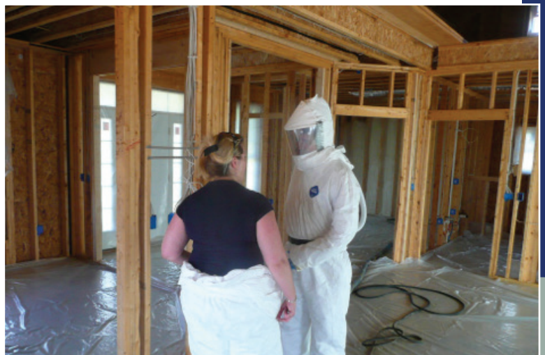
Figure 11: Provide notice to trades and occupants
