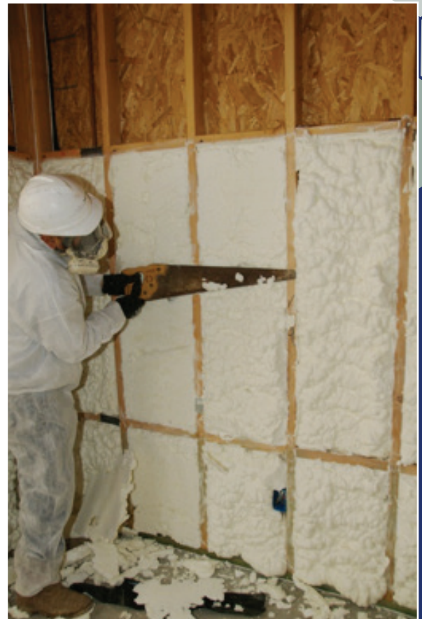
Figure 15: Contractor trimming foam
